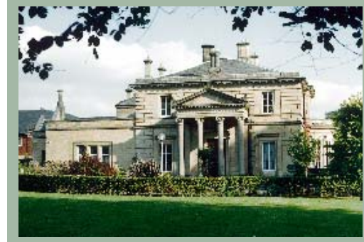
Spire Leeds Hospital
